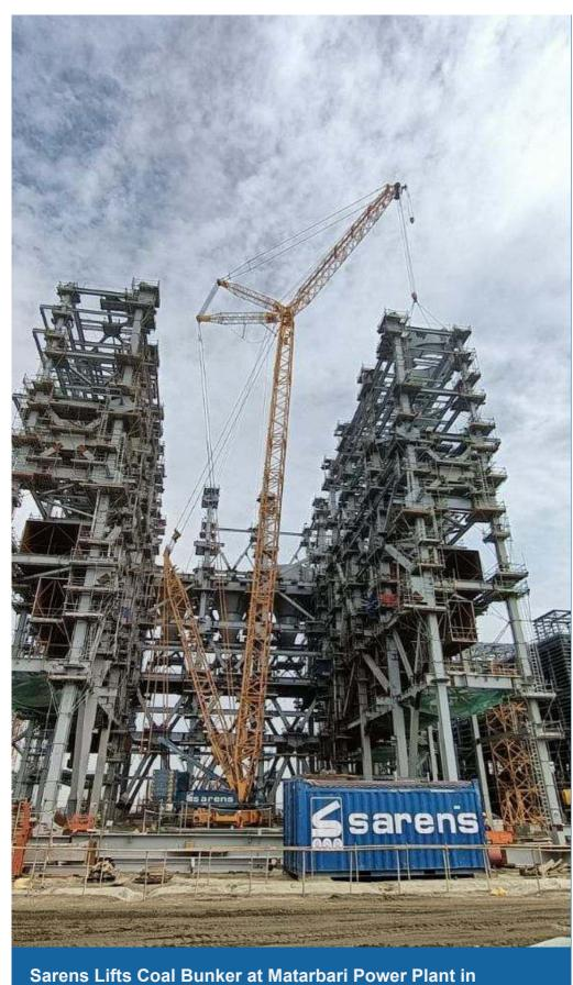
CC2800-1 crane lifts 70-tonne load during 10-month operation at the power plant.
